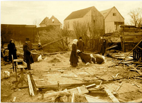
Farm on North Avenue Razed
